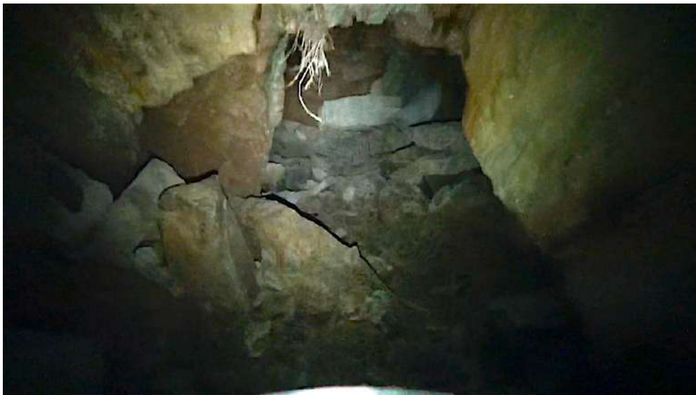
Tunnel turning to the left
